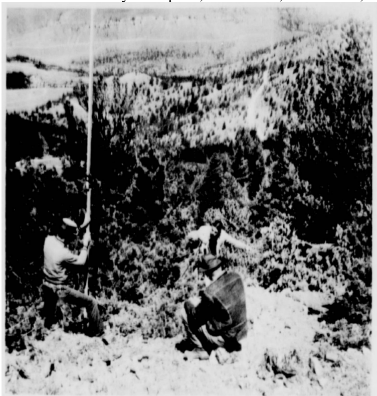
WORK WAS PROCEEDING ON SCHEDULE, despite the highly uneven terrain and strong winds on top of Dead Indian Hill, as Forest Service survey crews laid out the path of the new Cody to Sunlight Basin road. Above, Scott Tucker, Larry Hansel and Mike Smith work at staking levels for the new, wide and less dangerous road. When completed, the road down the slope of Dead Indian Hill to Dead Indian creek will be on an average 6% grade instead of the present 8 to 14% grade. The fifteen or twenty switchbacks curves will be reduced to five, with much wider radius. The entire new road will be twice as wide as the present. Work started out at progress of 2 miles a week, and is now down to about a mile a week due to the difficult timbered slopes. About six weeks is left on the survey job. —(Enterprise photo)
